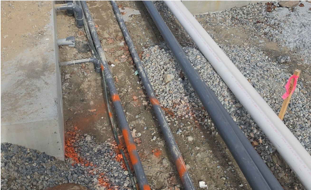
Underground conduit in the trench before it gets covered. If it is changed work, photograph it now.
